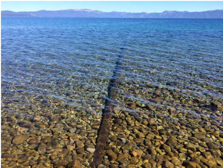
Photo 10: Existing Chambers Landing Intake Pipe - looking east.
