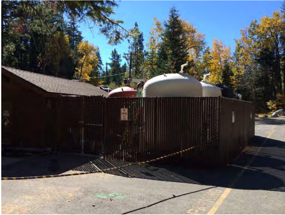
Photo 5: Existing Temporary WTP Site - looking west.
