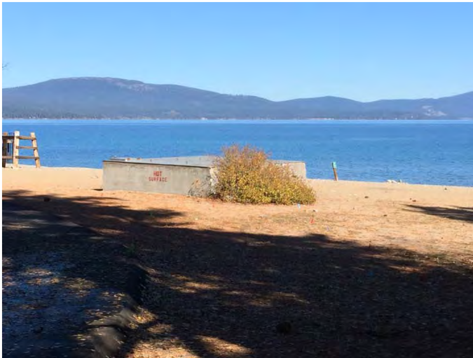
Photo 8: Existing Chambers Landing Intake - looking northeast.
