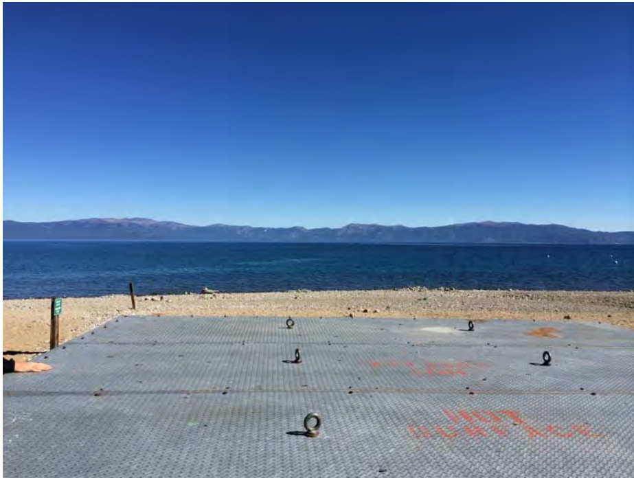
Photo 9: Existing Chambers Landing Intake - looking east.
